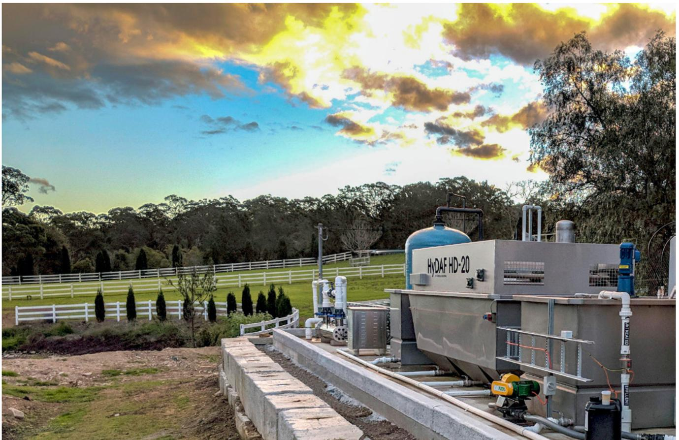
Chemical treatment combined with physical removal in a dissolved air flotation system provides an effective solution for removing phosphate in industrial wastewater, allowing the clean treated effluent to be safely discharged.
